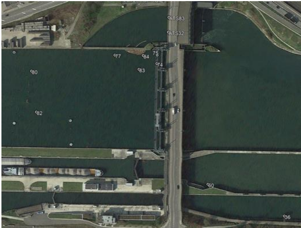
Figure 20 : view of the telemetric network installed at CH Ramet during the smolt 2021 survey.
