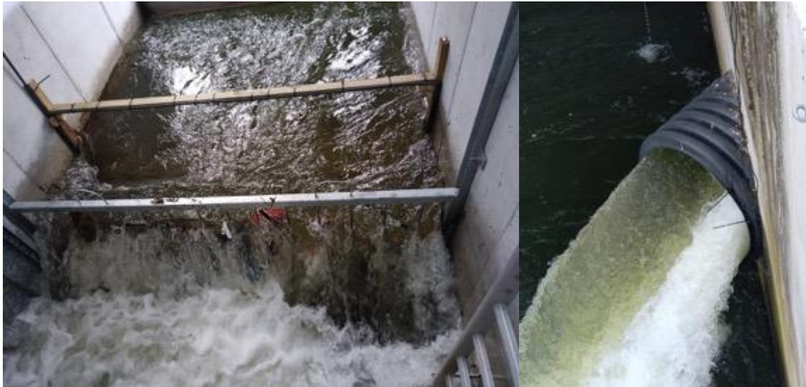
Figure 9 : view of the wooden frame in the upstream part of the bypass (left) and the cable around the outlet tube downstream (right).
