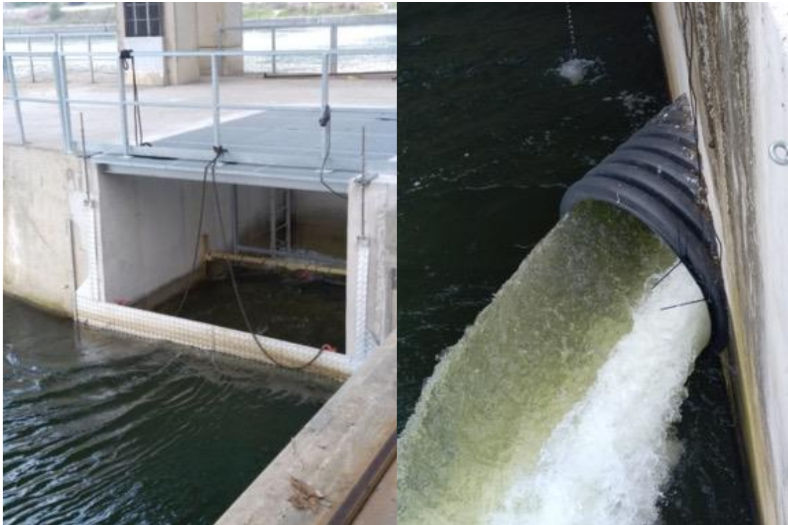
Figure 6 : pictures of the entrance (left) and outlet (right) of the bypass designed in CH Grands-Malades.
