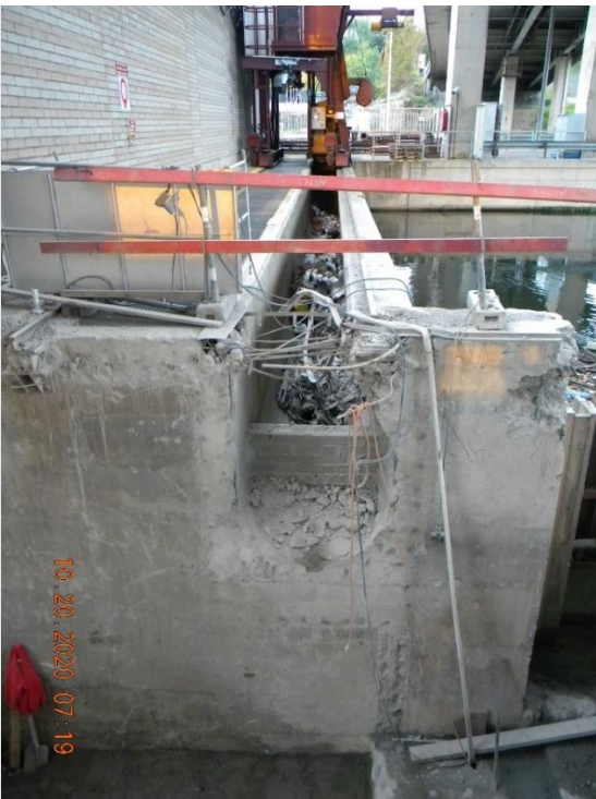
Figure 25 : demolition of the remaining concrete. Picture 3
