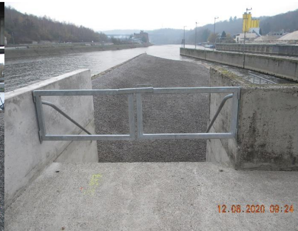
Figure 39 : View of the site after the end of the work. Picture 2
