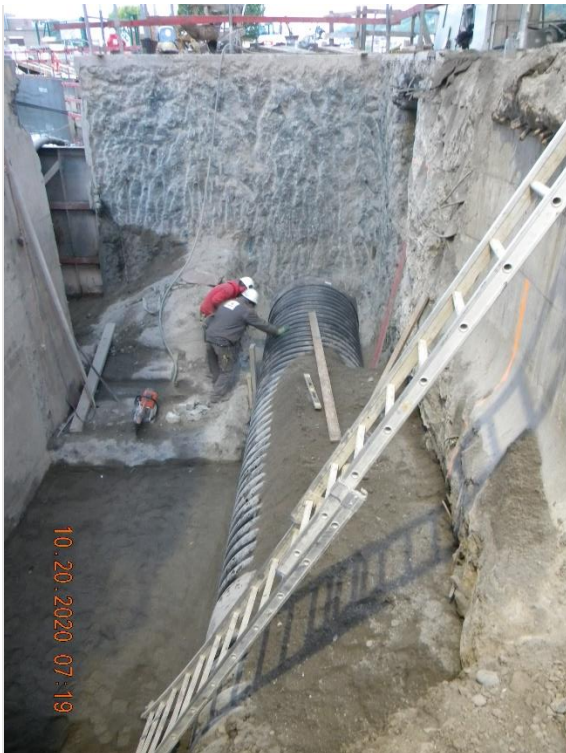
Figure 29 : Placement of the pipe (upstream). Picture 3
