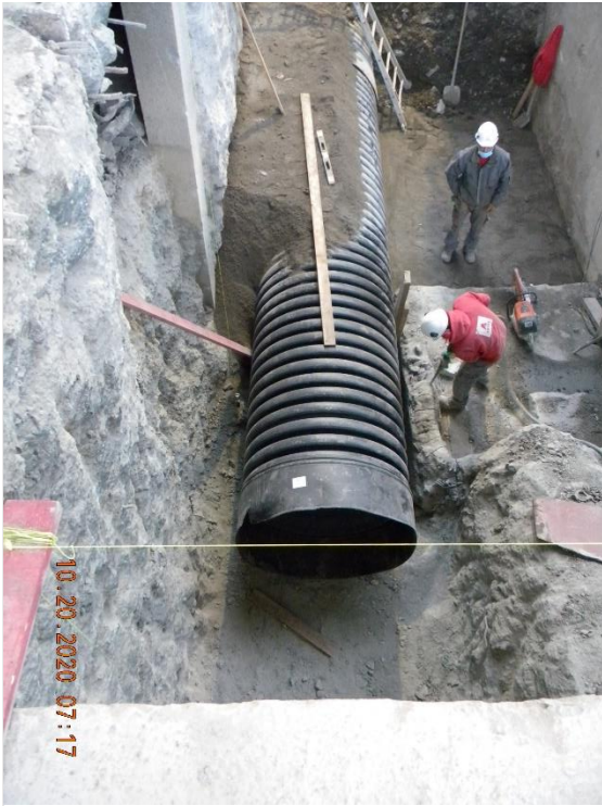
Figure 27 : Placement of the pipe (upstream). Picture 1
