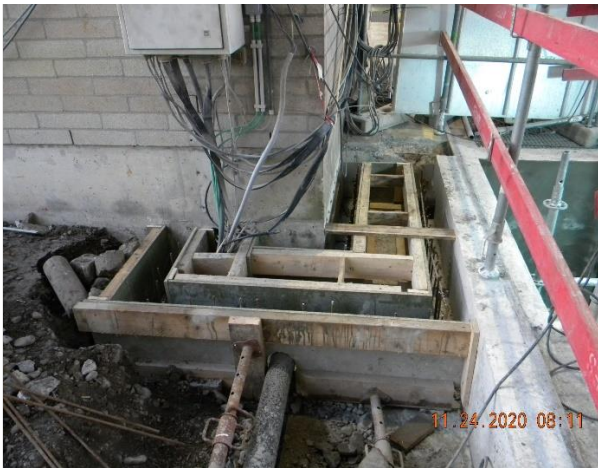
Figure 32 : placement of reinforcement. Picture 1
