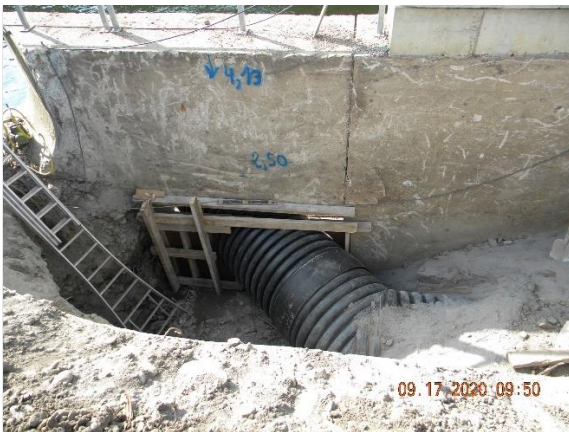
Figure 21 : View from above of the exit of the fish path. Picture 1
