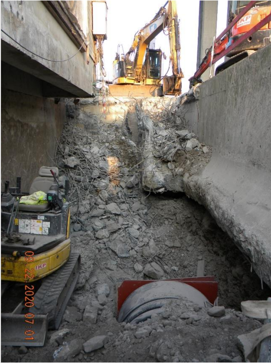
Figure 23 : demolition of the remaining concrete. Picture 1
