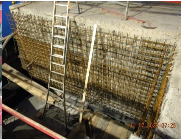
Figure 33 : placement of reinforcement. Picture 2
