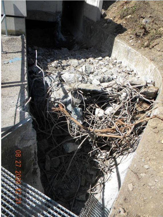
Figure 8 : demolition of the existing channel. Picture 1
