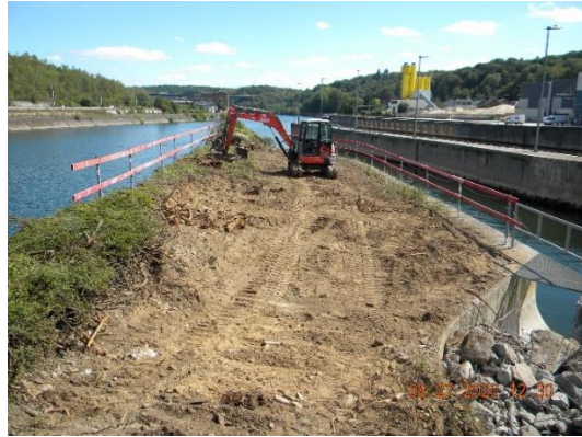
Figure 7 : Placement of the platform
