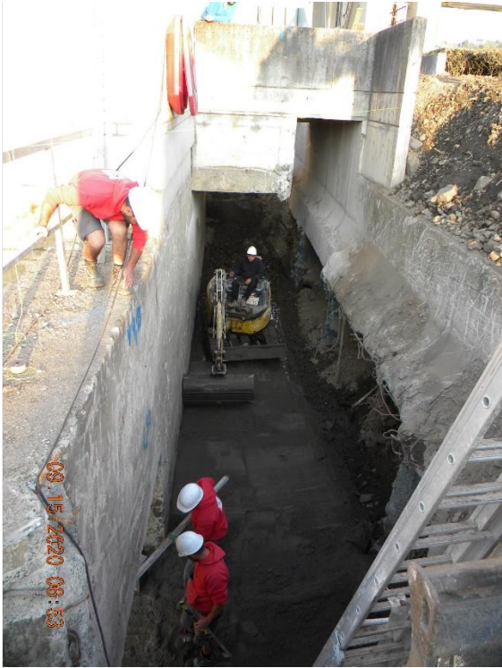
Figure 19 : Preparation of the support for the pipe. Picture 2
