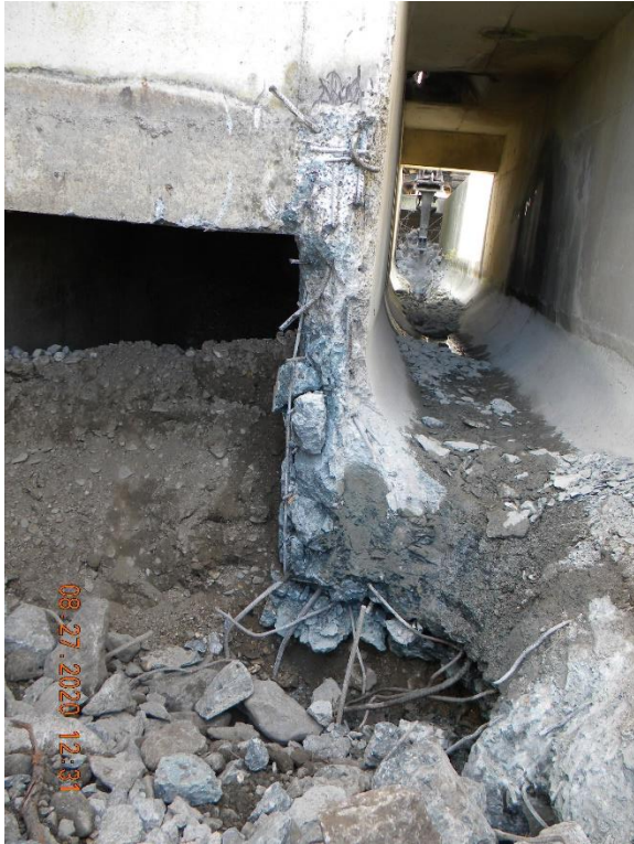
Figure 12 : demolition of the existing channel Picture 5
