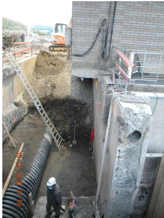
Figure 30 : Placement of the pipe (upstream). Picture 4
