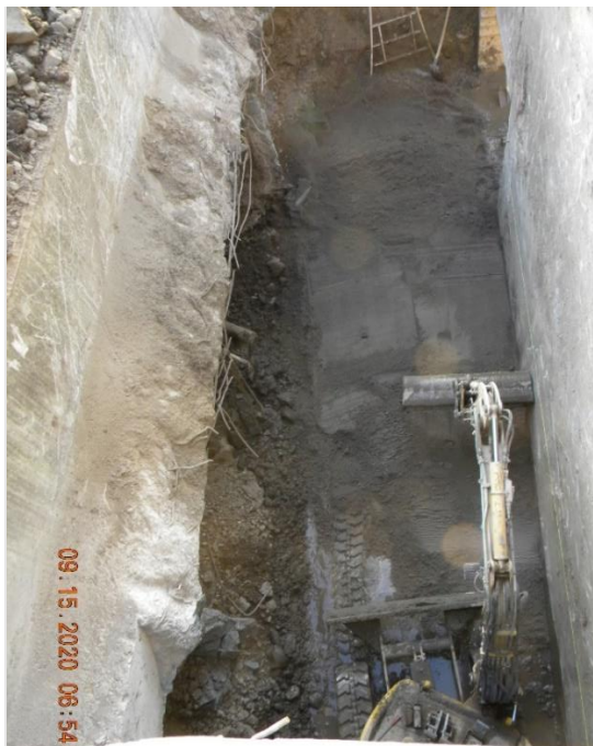
Figure 14 : Preparation of the support for the pipe. Picture 1
