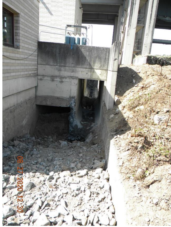
Figure 9 : demolition of the existing channel Picture 2
