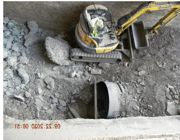
Figure 24 : demolition of the remaining concrete. Picture 2
