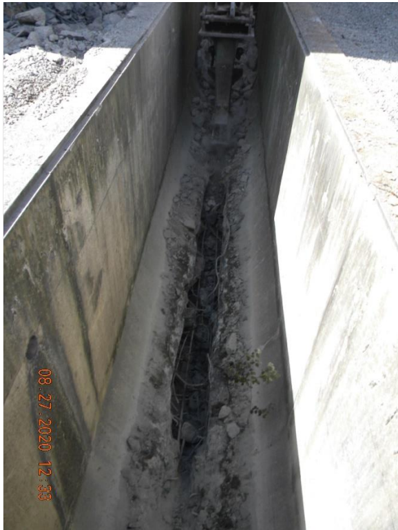
Figure 10 : demolition of the existing channel Picture 3
