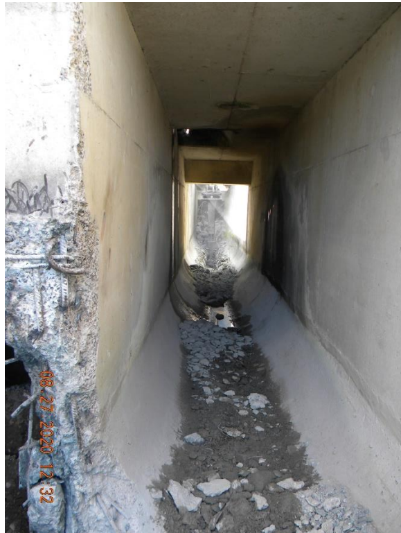
Figure 11 : demolition of the existing channel Picture 4
