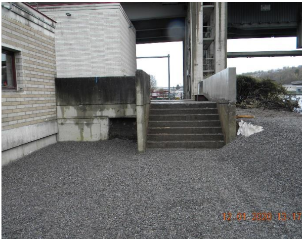
Figure 38 : View of the site after the end of the work. Picture 1
