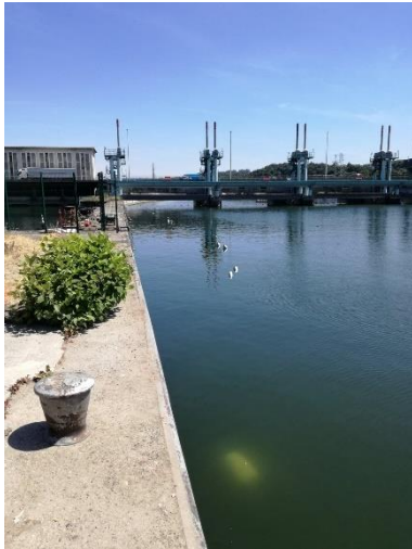
Figure 26 : Concrete block positioning
