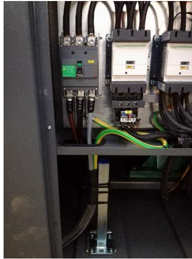
Figure 8 : Compressor electrical connection
