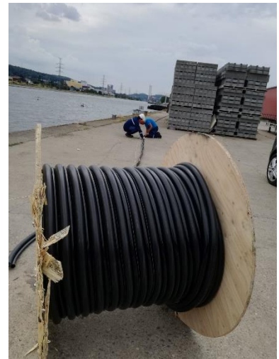
Figure 31 : Bubble pipe cutting
