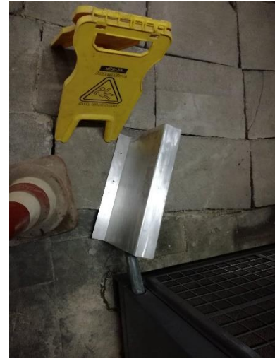
Figure 9 : Power supply protection
