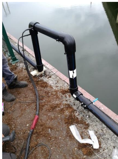
Figure 17 : Expansion loop
