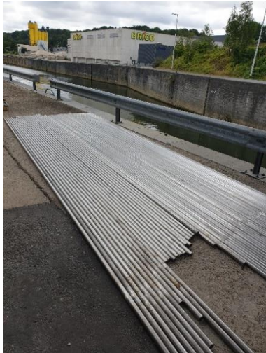
Figure 6 : The stainless steel pipes of the electrodes
