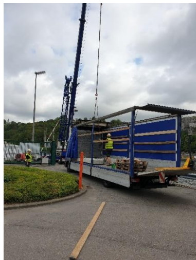
Figure 4 : The delivery truck with the concrete blocks
