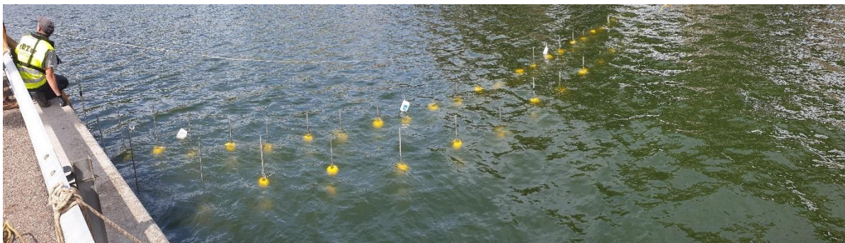
Figure 22 : The barrier after the first installation
