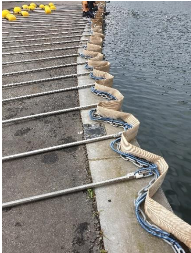
Figure 16 : The water hose before fixed on the chain
