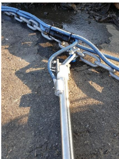
Figure 12 : The connection once the isolating product was put
