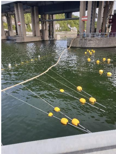
Figure 19 : The barrier and the inflated water hose
