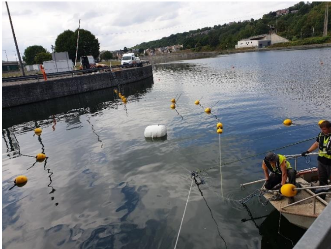
Figure 26 : The parachute and the hoist used to pull the chain out of the water
