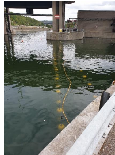
Figure 25 : The barrier after cutting of the electrodes
