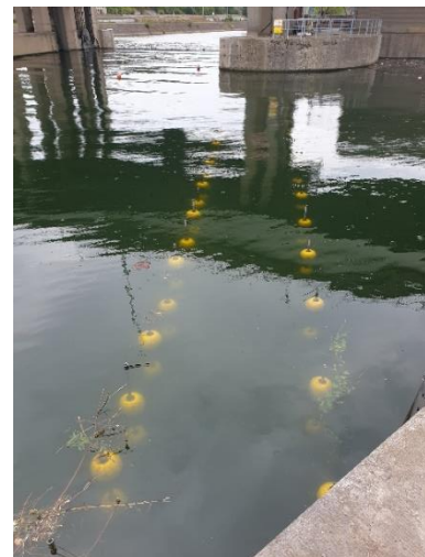
Figure 29 : The barrier before Procom came back to add some part to the shortest electrodes
