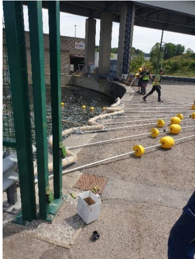
Figure 17 : The start of the installation of the barrier
