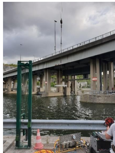
Figure 5 : A concrete block hold by the crane before the submersion
