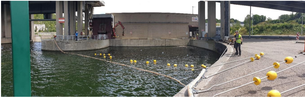
Figure 18 : The installation of the barrier
