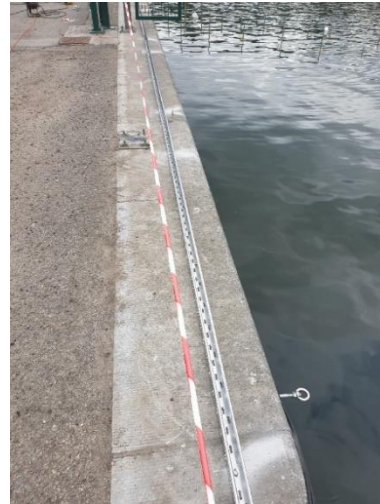
Figure 3 : The Railway cable
