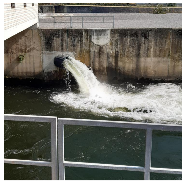
Outlet downstream of the power plant
