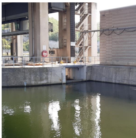
Outlet upstream of the power plant
