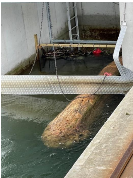
The blade couldn't resist to trunks
