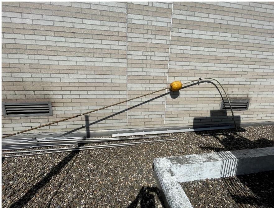
Electrode number 5 twisted probably by the trash cleaner
